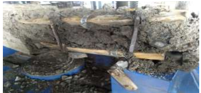
Fig.5 (Bamboo Reinforced Beam)
