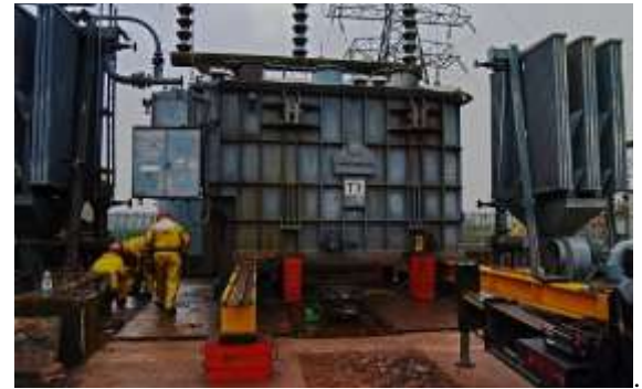
Fig2: Cleaning of Transformer
