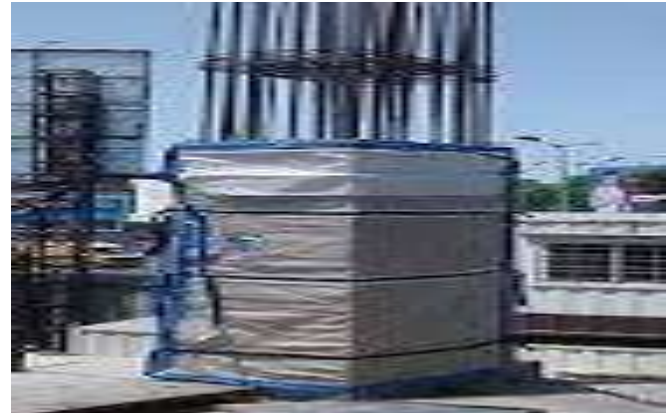
Fig-4: Curing by Drip
