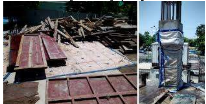
Fig-5: Curing by Drip
