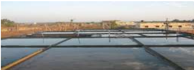
Fig-1: Curing by ponding
