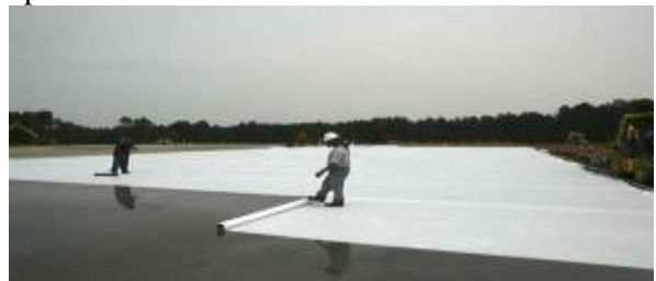
Fig-3: Curing by impervious paper
