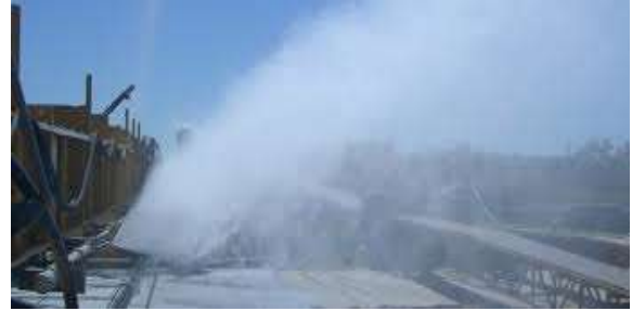
Fig-2: Curing by Fogging
