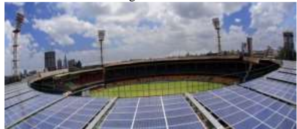
Fig.(ii) : Solar Plant in M. Chinnaswamy Stadium, Bangalore.
