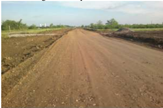
Fig. 2: Soil Road After Applying Terrazyme
