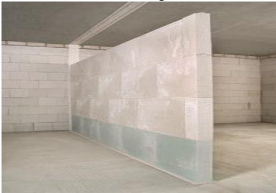
Fig. 3: Construction of a non-load bearing partition wall of Gypsum Blocks
