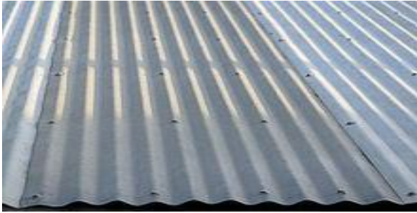
Fig5: Corrugated Fibre cement roofing
