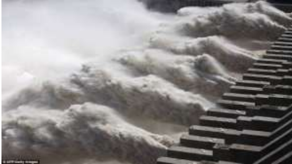
Figure 4: flooded water discharges through the spillway
