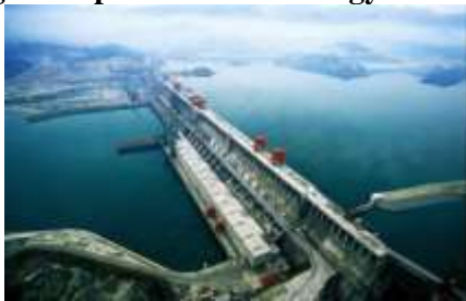
Figure 2: picture of the three gorges dam
