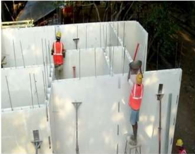
Fig-4: Concrete filling in GFRG panel
