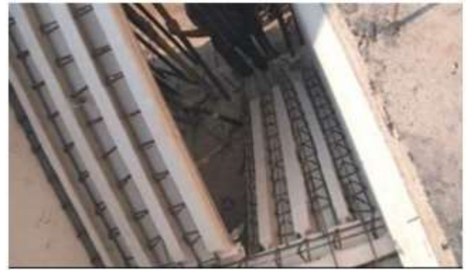
Fig-6: Reinforcement for concealed beams in waist slab
