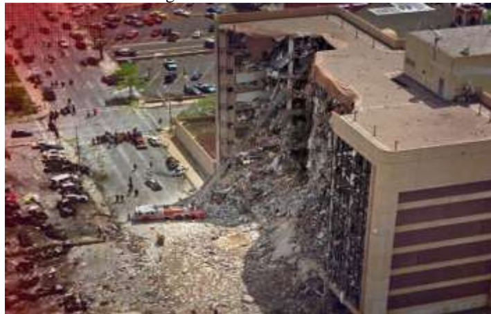
Figure 5. Original Image of Federal Building after Blast.
