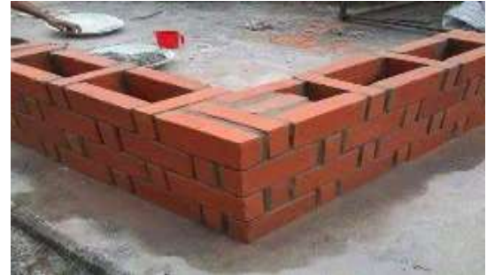
Fig-4: Corner joint in Rat trap bond
